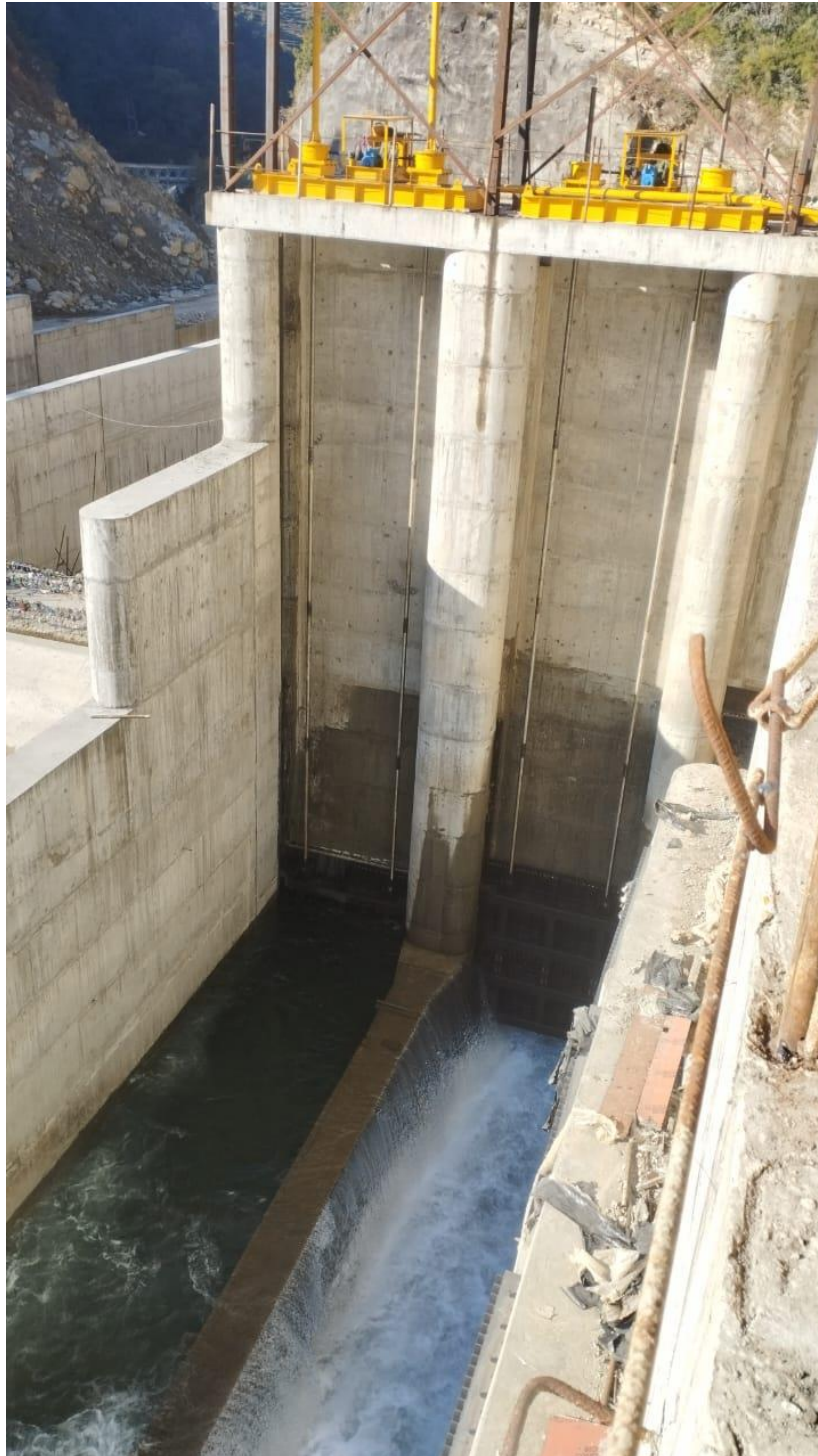
Figure Under Sluice Gate
