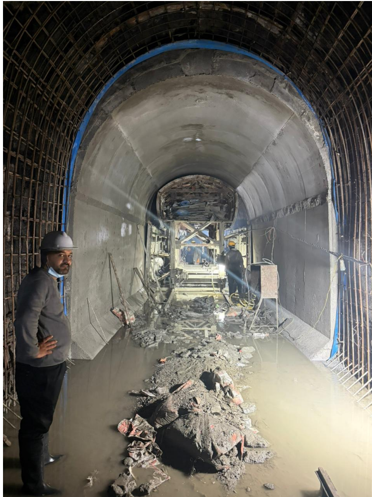
Full Concrete work in Face 3
