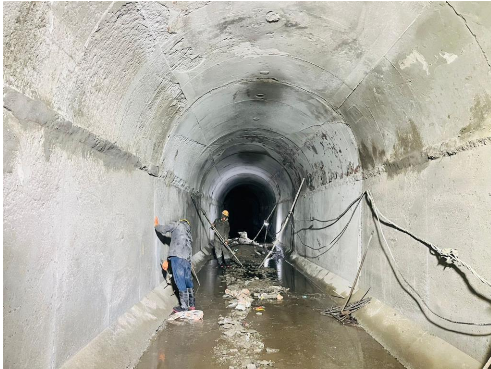
Face 2: Full lining work in face 2 completed
