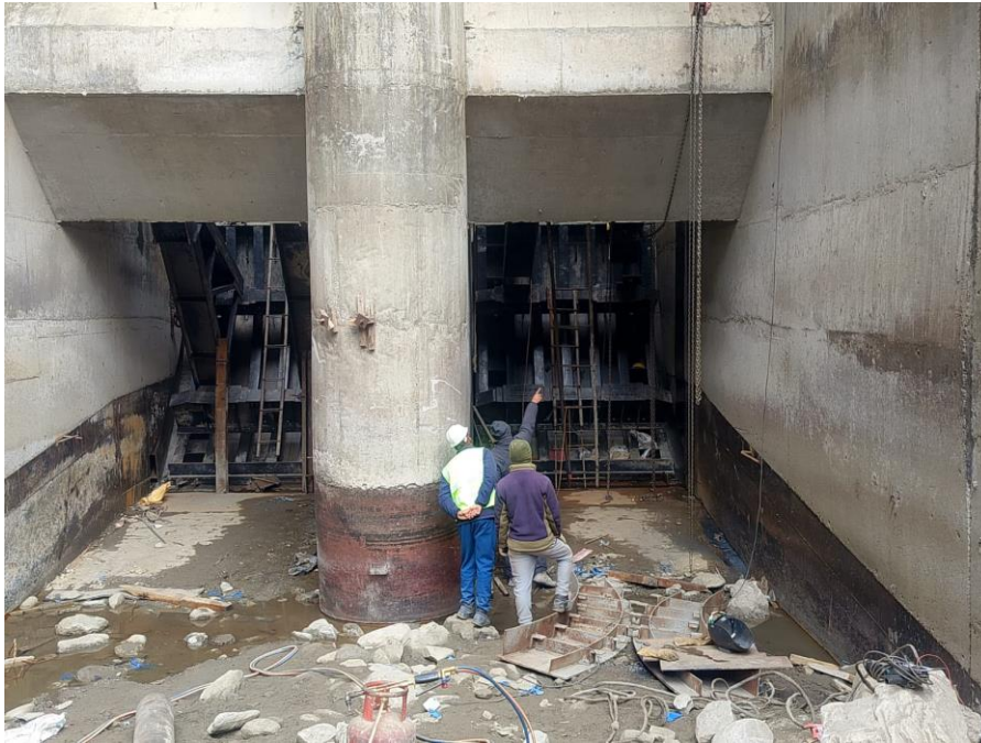
Installation of the Radial Gate at headworks
