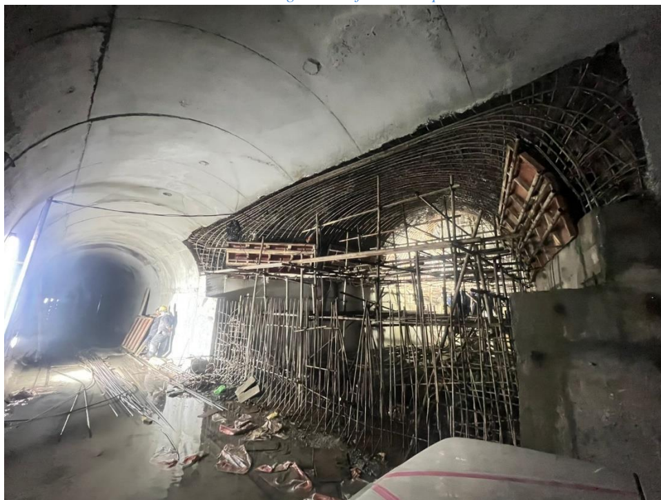
Face 2: Phulping brook shaft junction formworks continue
