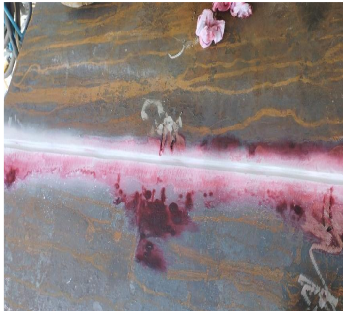
DPT testing in joints
