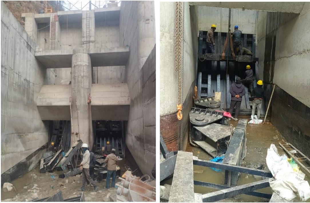
Preparation for the installation of the radial gate
