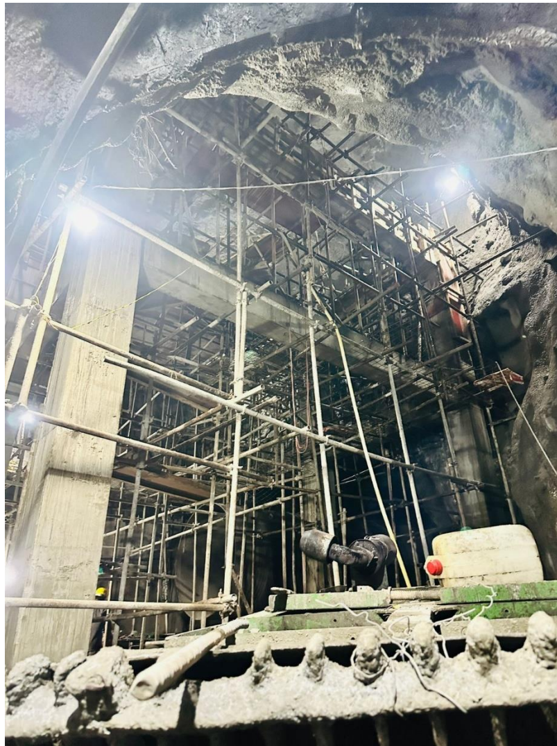
Valve Chamber Work at Valve House
