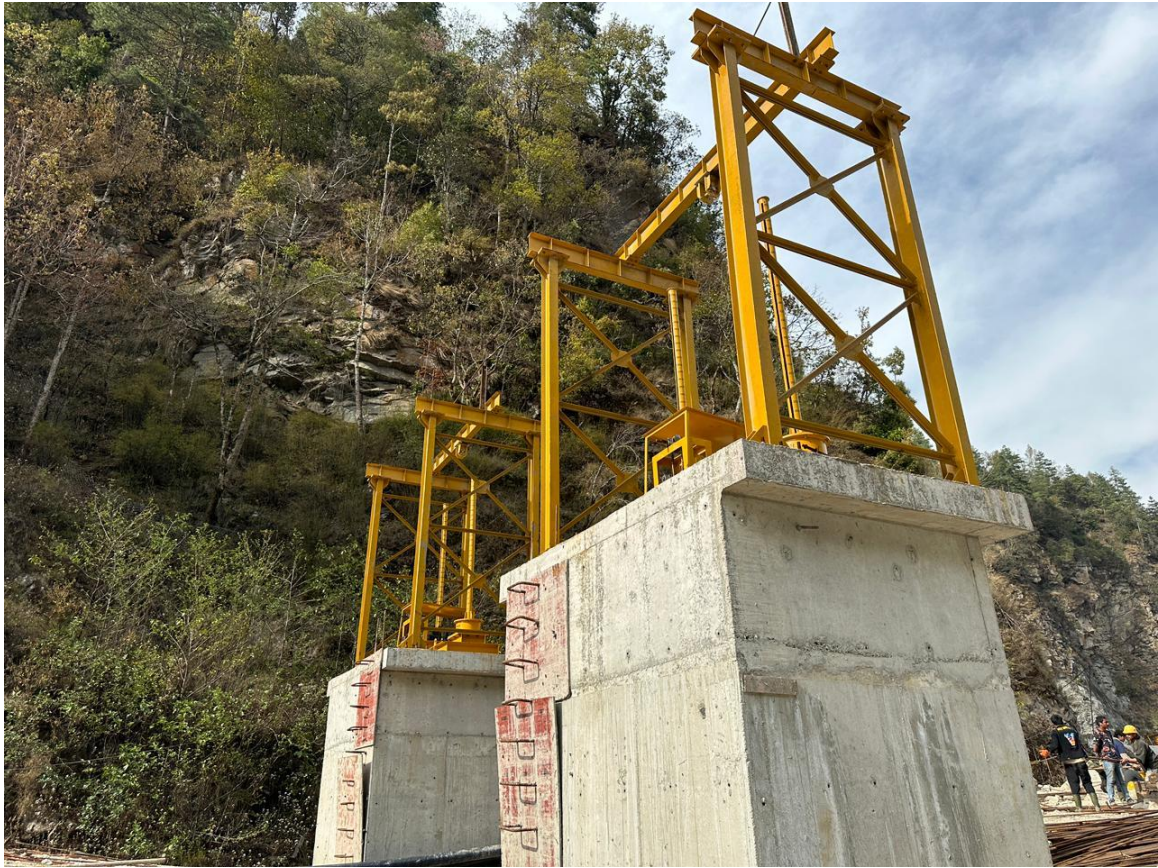
Hosting Installation of Gate
