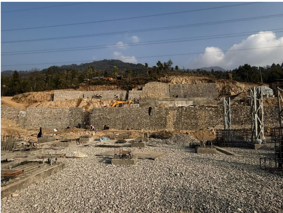
Masonry Work at LILO
