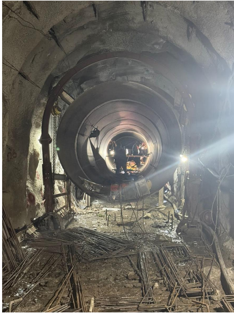
Pipe Installation work at UPT
