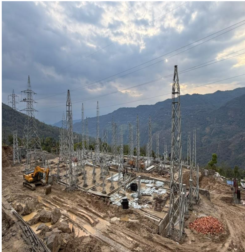
Substation steel structure erection on progressing
