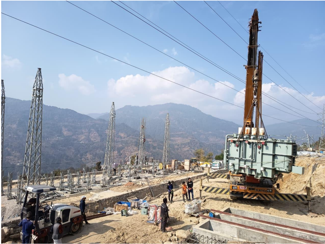
EM Structure Erection Work at LILO
