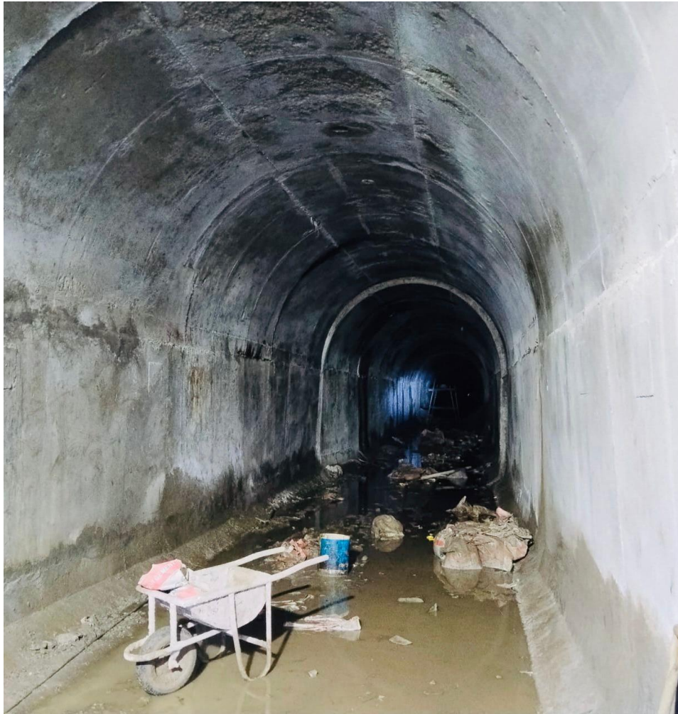
Concrete lining work in Face 1.
