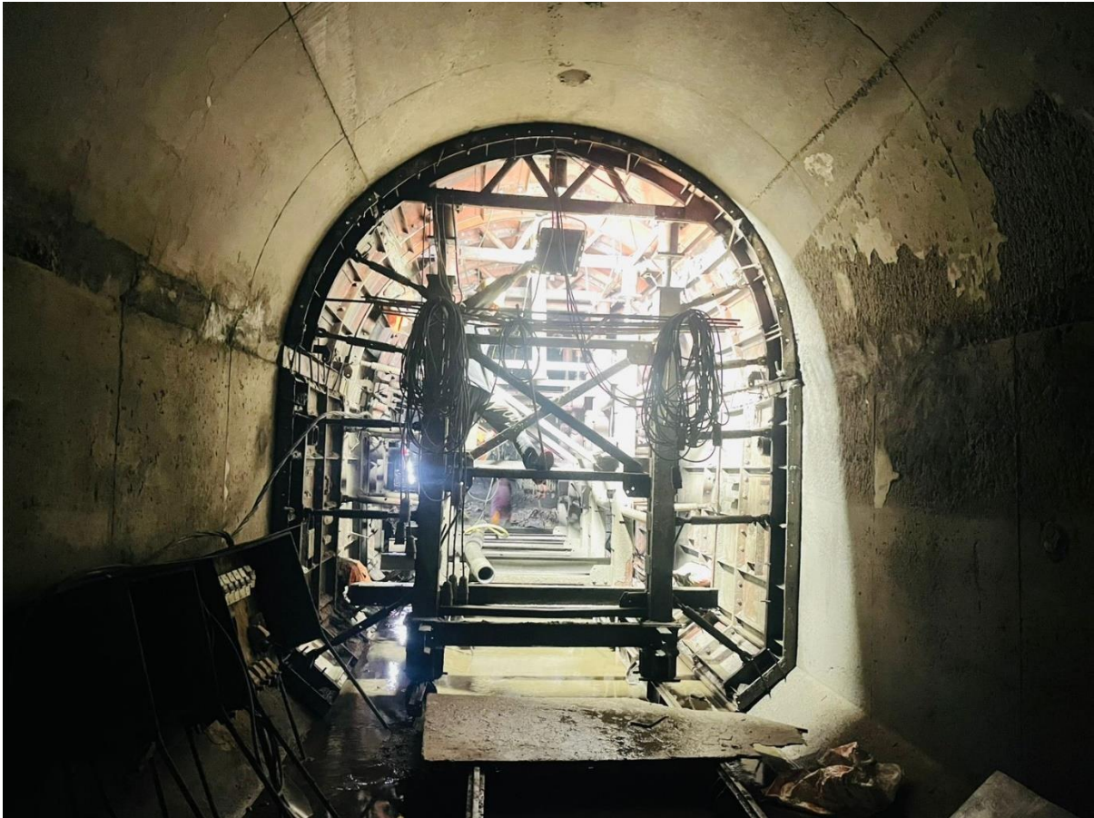
Gantry Preparation for the lining work in Face 1
