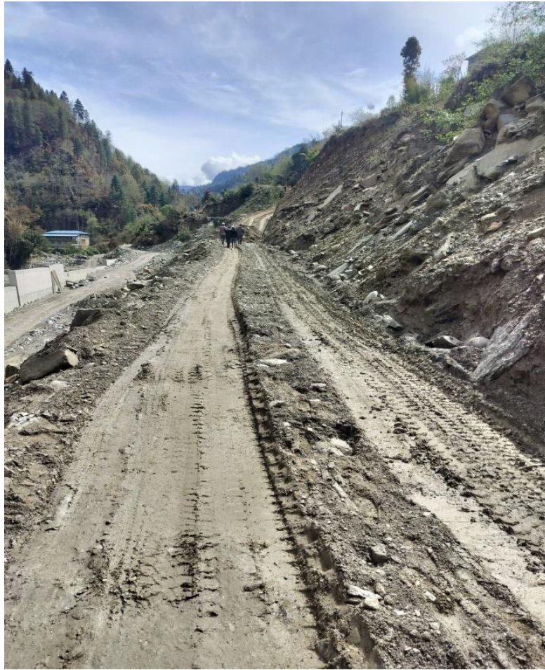
Back fill work along left bank
