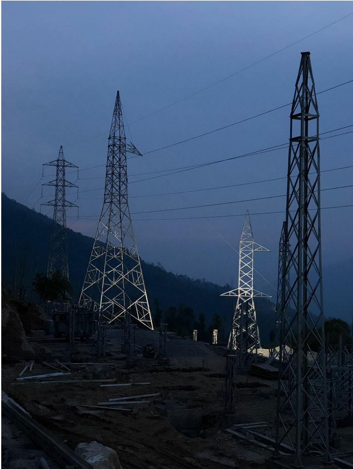
Incoming and outgoing dead end towers erection
