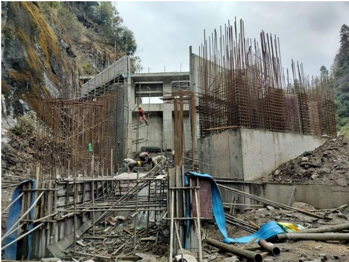
Inlet transition portion
